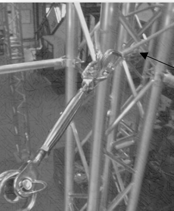
Picture 1 : Put sling around the anchorage
